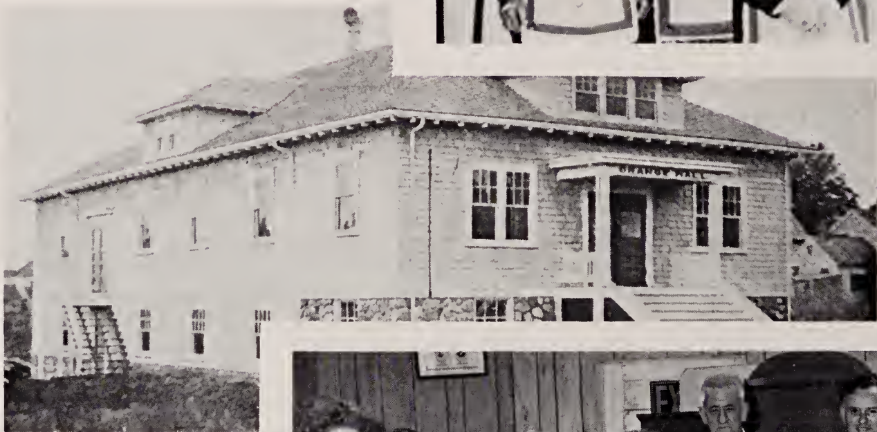
Grange Hall built in 1911
